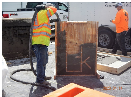
Concrete forming and pumping demonstration.
